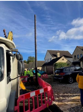
One of the 4 Poles installed by Full Fibre Ltd prior to them halting further work
